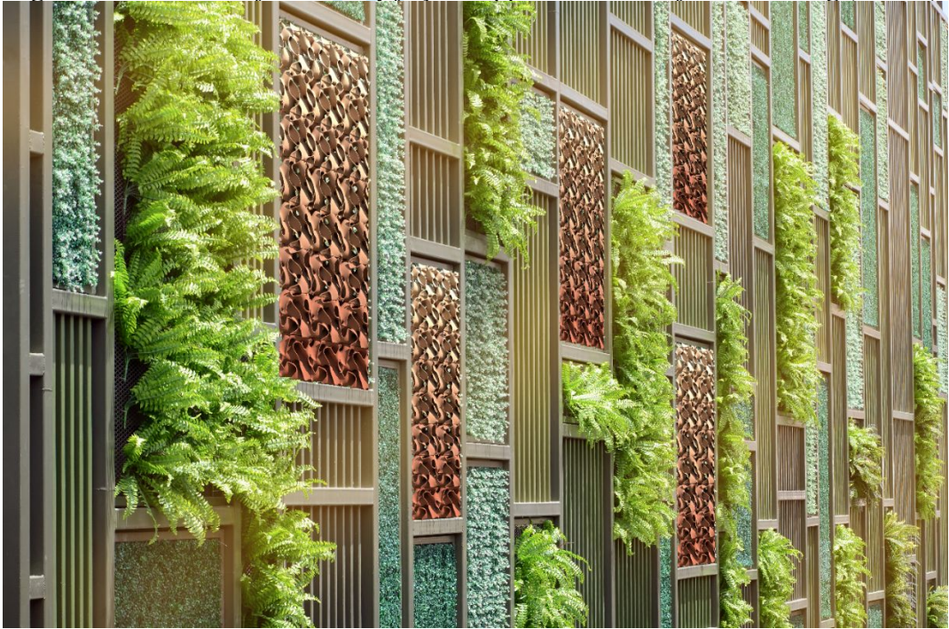
Figure 11. AeroTerra is applied to outdoor retrofit façades, serving as a secondary skin for the building.
